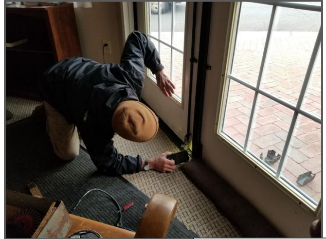
Tom Snarr working on the front door
